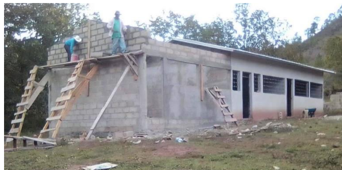
The third classroom of the new middle school under construction.
